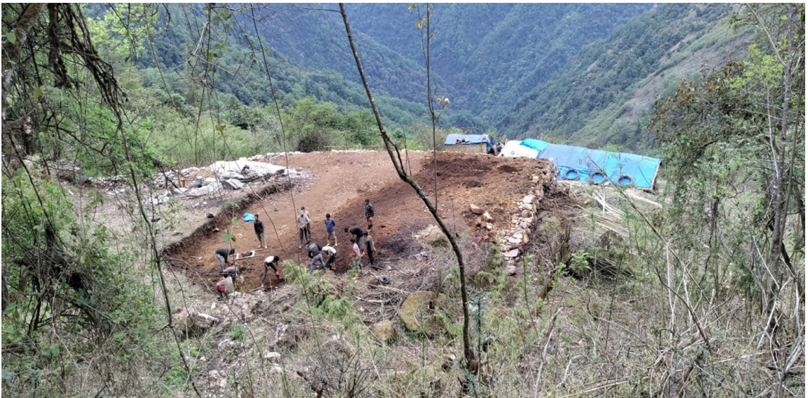
Construction of Survey Camp
