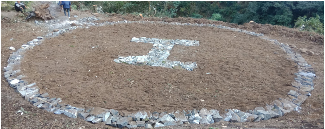
Constructed Helipad in Project Site
